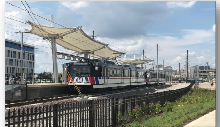
Cortex Metro Station 2018
